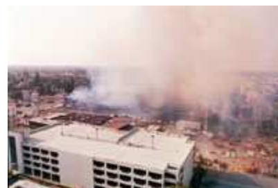
Aerial view of the Santana Row Fire.
